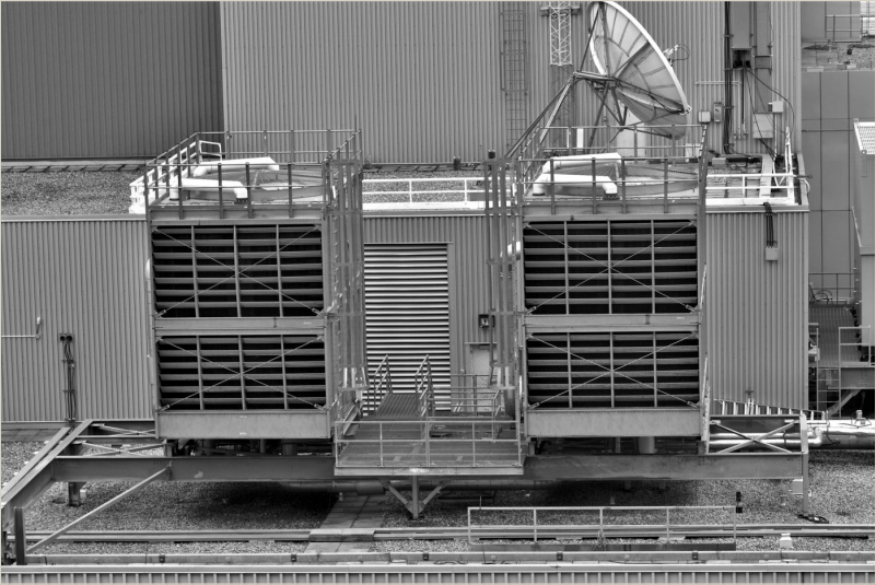
ROOFTOP COOLING TOWER INSTALLATION
