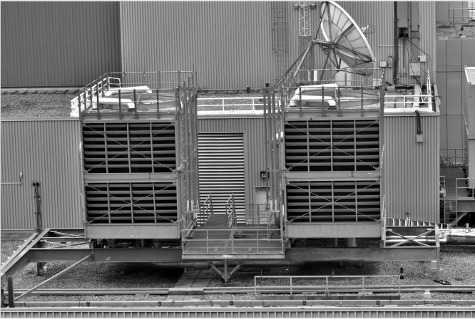
ROOFTOP COOLING TOWER INSTALLATION
