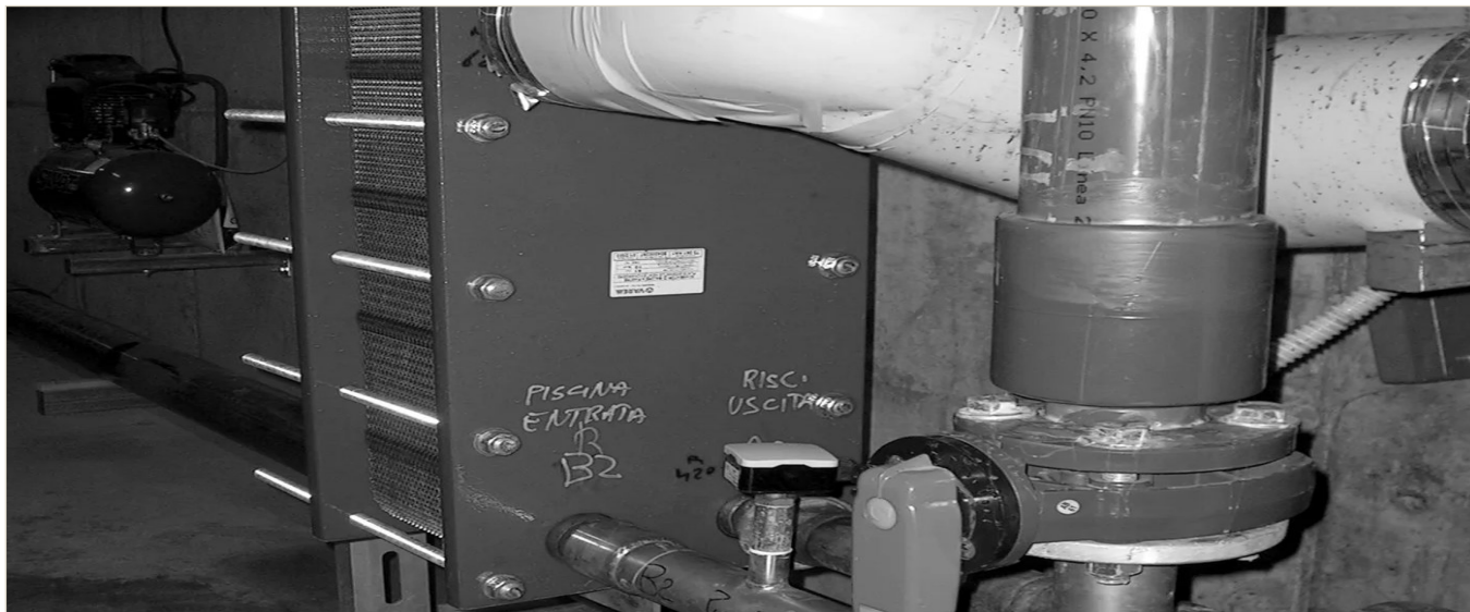
PLATE HEAT EXCHANGER / SERVICEABLE FRAME
