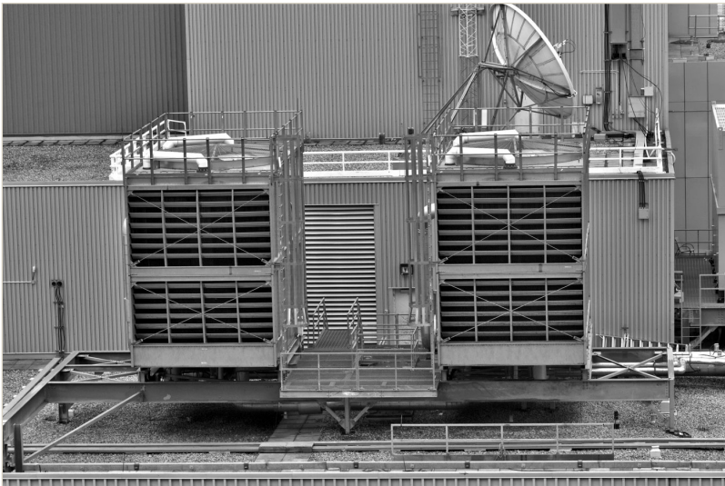
ROOFTOP COOLING TOWER INSTALLATION
