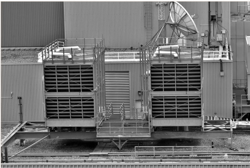
ROOFTOP COOLING TOWER INSTALLATION
