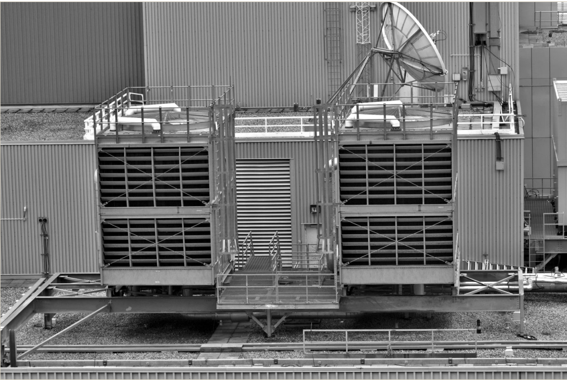
HYBRID COOLERS – REPRESENTATIVE NOVARYN EQUIPMENT
