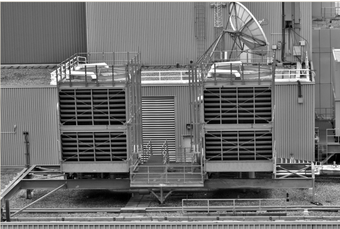
HYBRID COOLERS – REPRESENTATIVE NOVARYN EQUIPMENT
